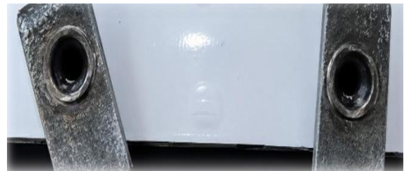
Figure 8 - Clip Nuts Installed
